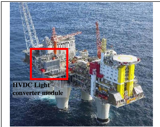
Figure 7: Troll A platform with HVDC Light® converter module
